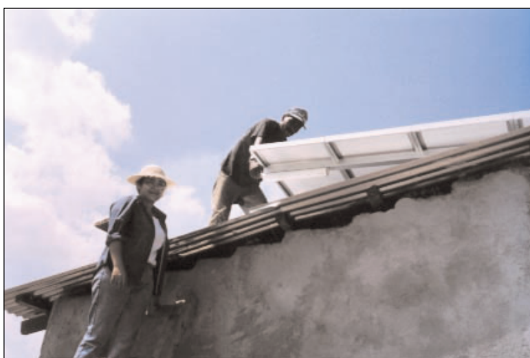
Figure 1 Technicians mounting array
